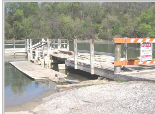
During the 2008 flood, the Kiwanis Pond fishing pier was destroyed by the high ground water level. This pier was a unique feature for Janesville in that it was originally donated in 1993 by the Janesville Kiwanis clubs and included handicap accessibility and unique fishing extending 60' from shore into 16' feet of water.
